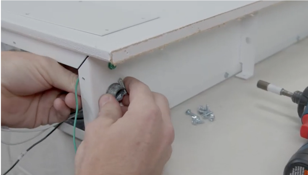
Figure 11 – Install the MC connector
