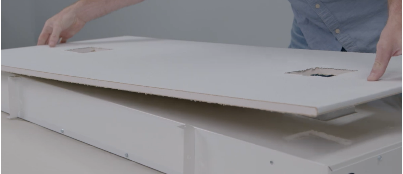
Figure 5 – Place cut tile onto fixture
