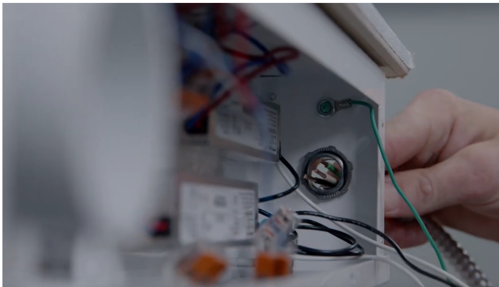
Figure 12 – Run the input wires through the MC connector opening
