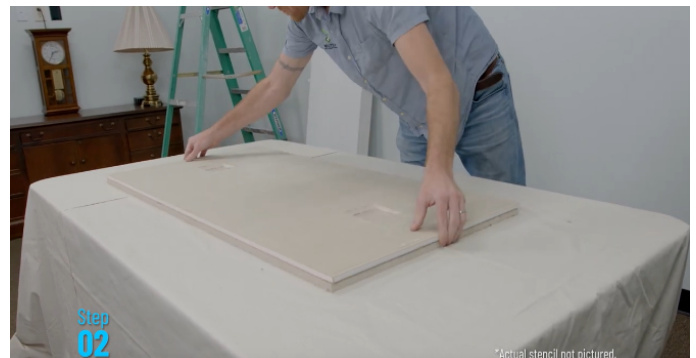
Figure 2 – Align installation template to tile
