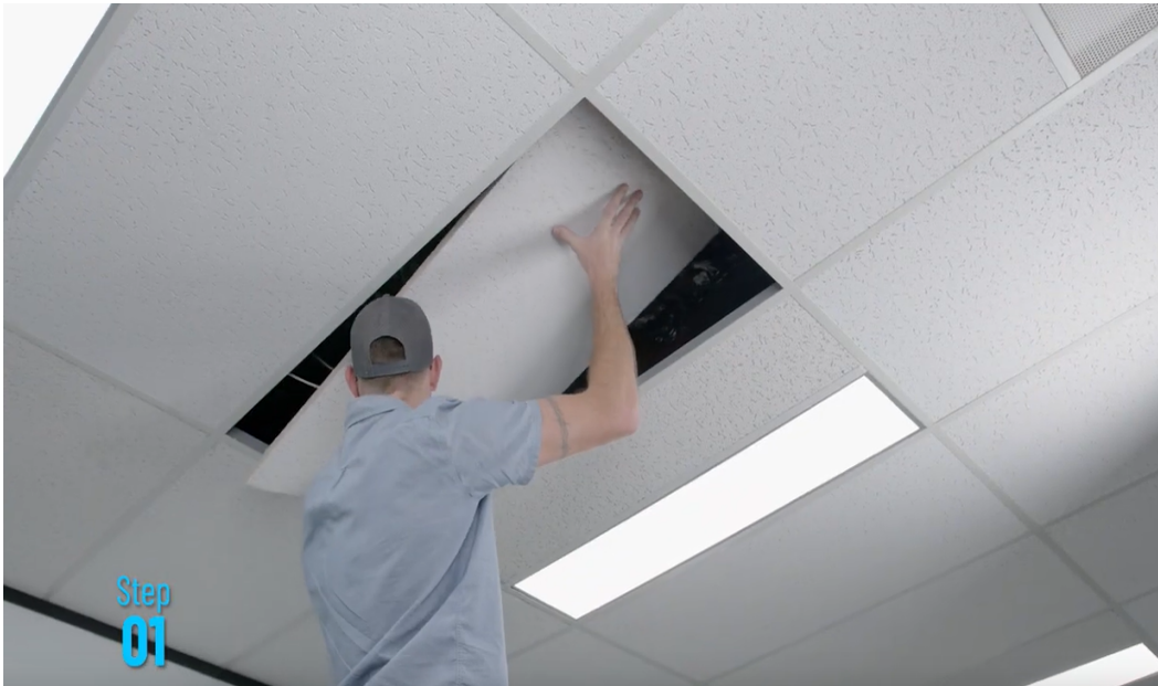
Figure 1 – Remove ceiling tile from grid
