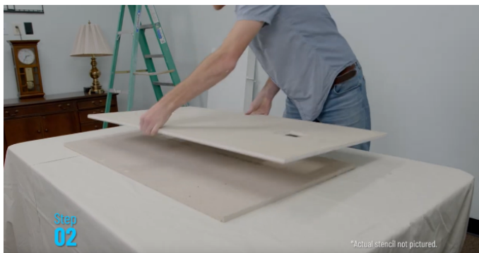
Figure 2 – Align installation template to tile
