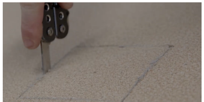
Figure 4 – Score and cut out intake hole(s)
