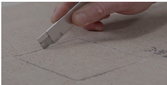
Figure 4 – Score and cut out intake hole(s)
