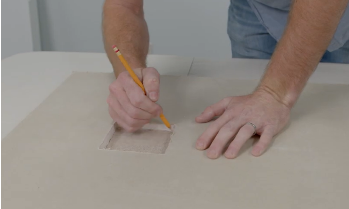
Figure 3 – Mark locations of intake holes to be cut
